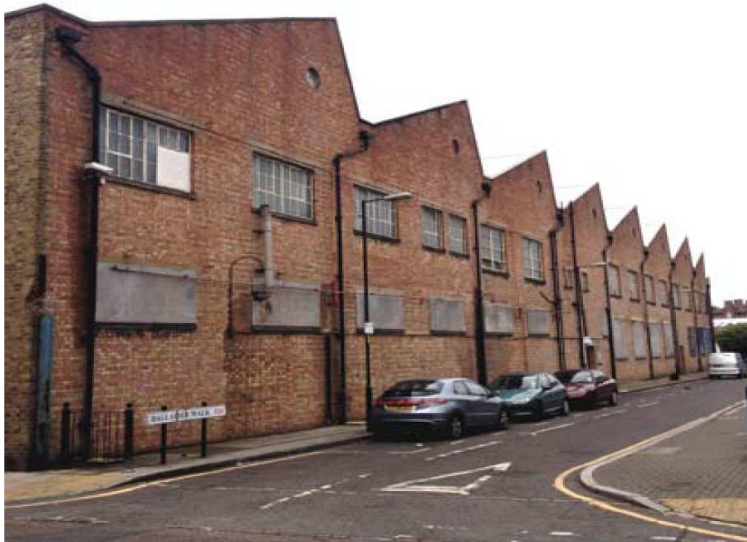
View along Balladier Walk showing 1939 factory building.
